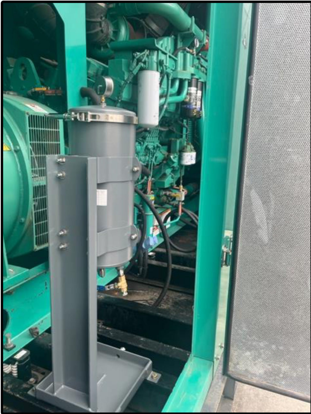
Backside of the HD-601 PetroSavers refiner unit on base mounting
