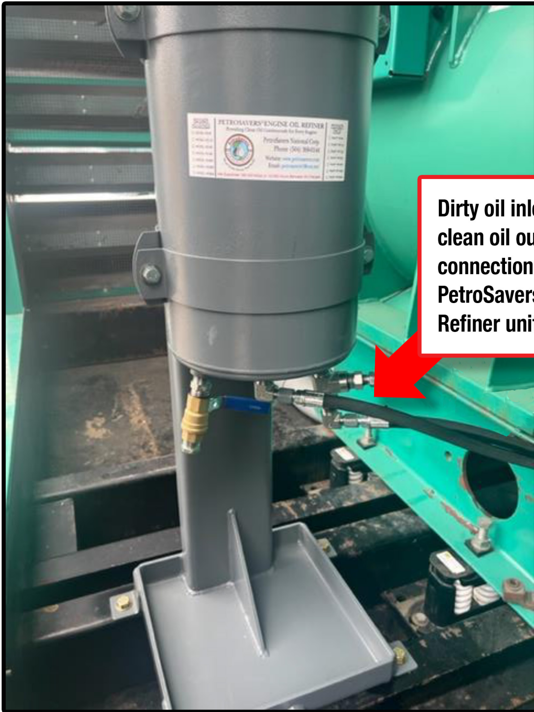
Inlet and Outlet oil line connections on PetroSavers unit.
